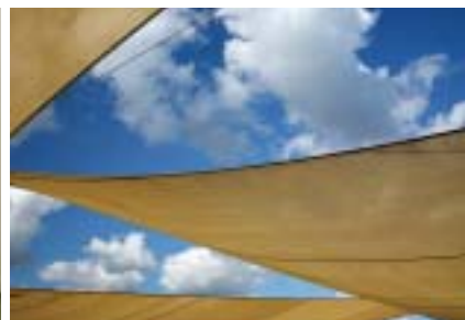
Removable shade sails allow winter sun whilst providing protection from summer sun. (Source: Your Home Technical Manual)
