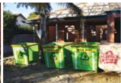
Tidy building site using EarthCare bins.
