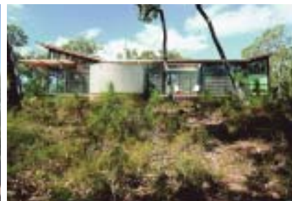
Example of lightly framed bush dwelling featuring extensive use of glazing steel water tank as a wall element. (Source: Richard Szklarz Architects)
