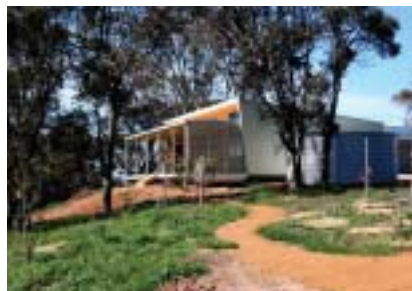
Example of single storey framed house sitting above the natural gradient with outdoor living area located to take advantage of views. (Source: Nordic Homes)
