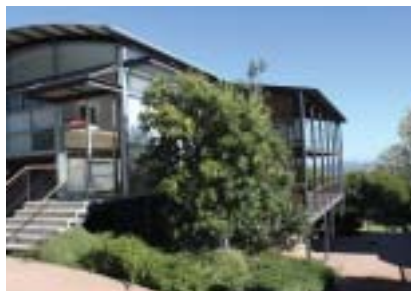
Built form example featuring vaulted roof, use of site gradient for parking and storage beneath the house.
