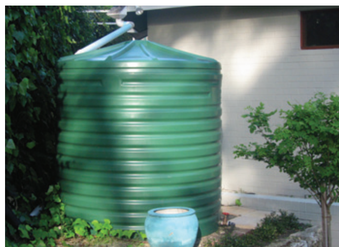
Example of rainwater tank provided to residents at Avon Ridge
